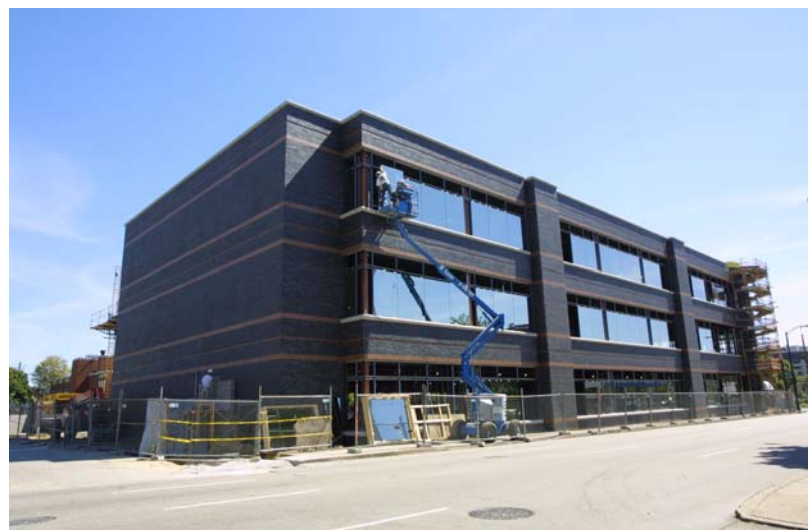
Business incubator under construction
